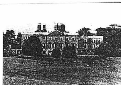
Copped Hall: the derelict mansion.
